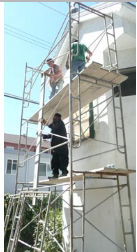
Установка лѣсовъ. Scaffold assembly.
